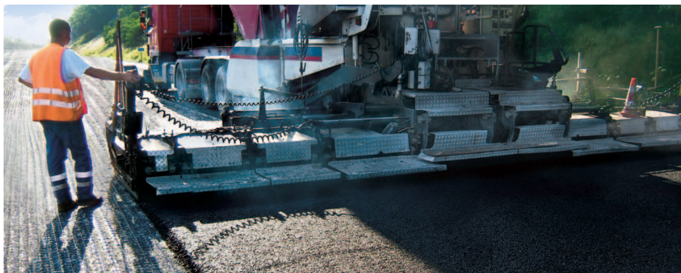
Paving takes place directly over the Tensar AR-GN.
