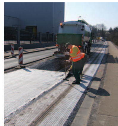
A simple overlap joint for Tensar Glasstex.
