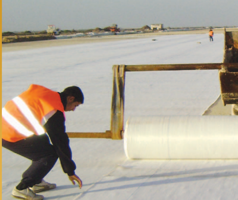
Tensor® Basetex™ geotextile installation at Oran airport in Algeria providing cost-effective installation and offering permanent high strength reinforcement below the fill layer.
