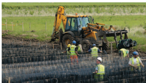
TensorTech® Stratum Foundation Mattress System is used here to control differential settlement over variable ground.
